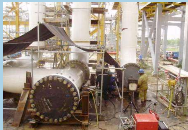
Hydrotest for Tie In Pipe Spool G17e/G18e (completed)
