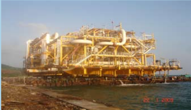
Load Out SMP Deck 22-01-2009
