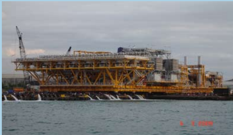
Load Out SCP Deck 04-03-2009
